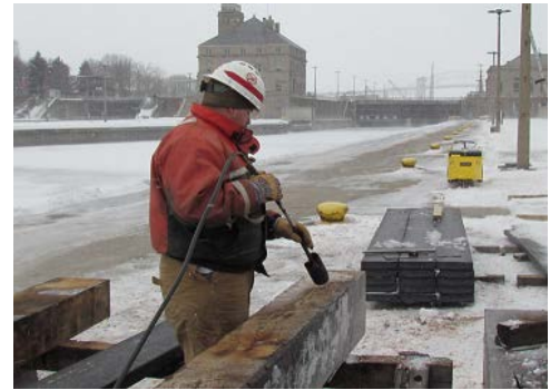
Image courtesy USACE Sault Sainte Marie, Ice Fender Repair at Soo Locks, 2012
